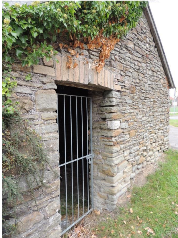
Plate 15. Gated entrance to chapel hut.
